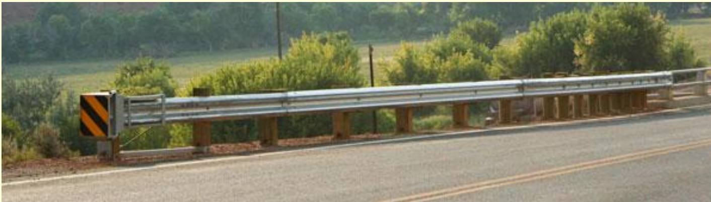
W-Beam w/ end section
