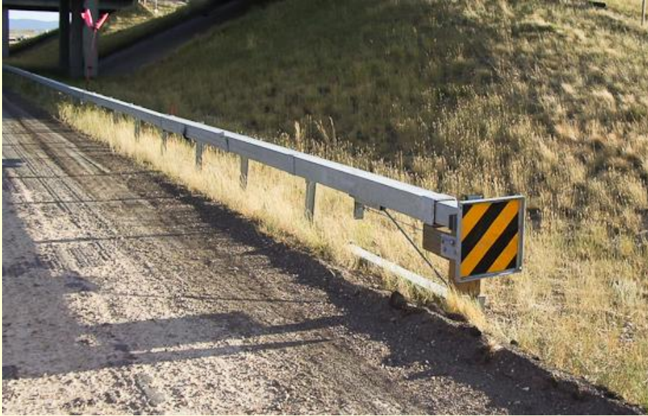
Box Beam w/ end section
